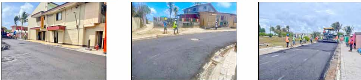
Newly asphalt paved roads.
